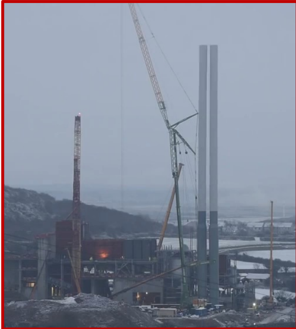
Twin chimneys (Cornwall, 2015)
